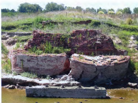
Fig. 11.3 Massive construction of brick and wood at the southern end of the Salado Bridge, exposed by the low river level in 2009
