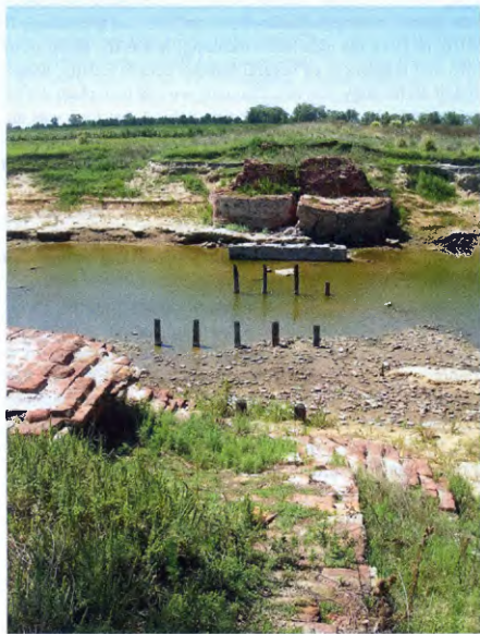
Fig. 11.1 Remains of the Salado Bridge when the river was at an unusually low level in 2009. The pillars in the water that helped its construction and support are still visible
