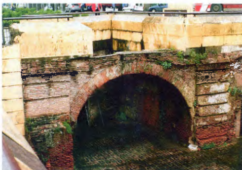
Fig. 11.6 Archaeological remains of the tunnels which run inside the Customs Central Building, built to accommodate the differences in level between the river and the city, excavated in 1983–85
